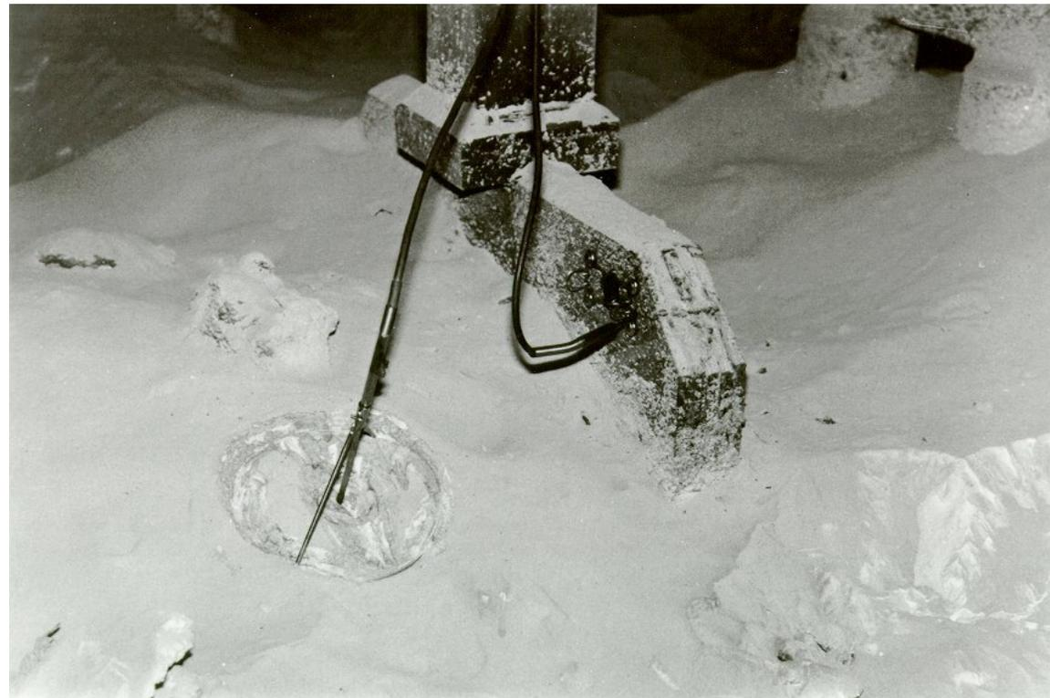
Measurement of the heat flux on the crust and the anode yoke using Japanese heat flux probes in the 70's
